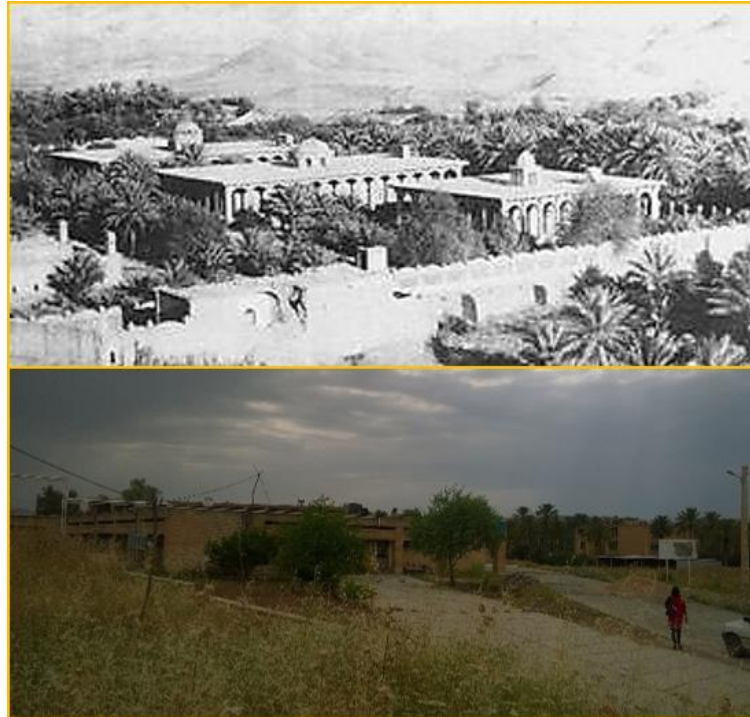
Fig 4. Comparison between pre- and post-war condition of Quarantine Hospital Top: before the war [16]; Bottom: after the reconstruction, (Source author, 2016)
