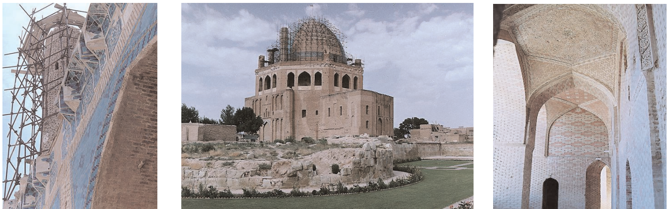
Fig. 6. Photographs of Gunbad-i-Sultaniya (Oljeito Mausoleum), presented in the sheet of "Structural value"
