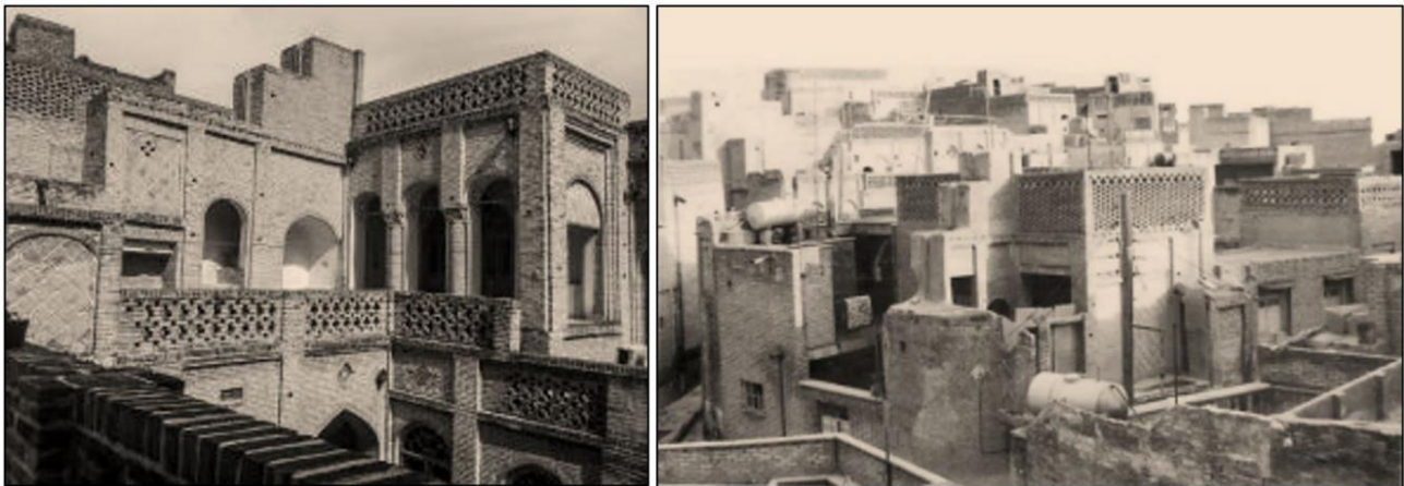
Fig 16. The Reverse Application of Lattice in the Roofs of the Buildings (Source: Authors)
