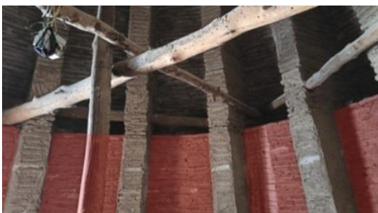
Fig 12. Increasing the Thickness of the Drum in the Panje Shah Tomb
