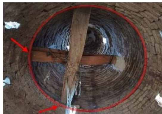
Fig 10. The Reduction of Thickness in the Cheheltan Tomb
