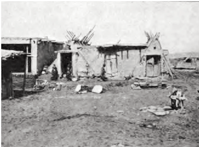
Fig. 3 Extended model of “A shaped” shelters consist of 2 tent-models bridged with a flat roof [11]
