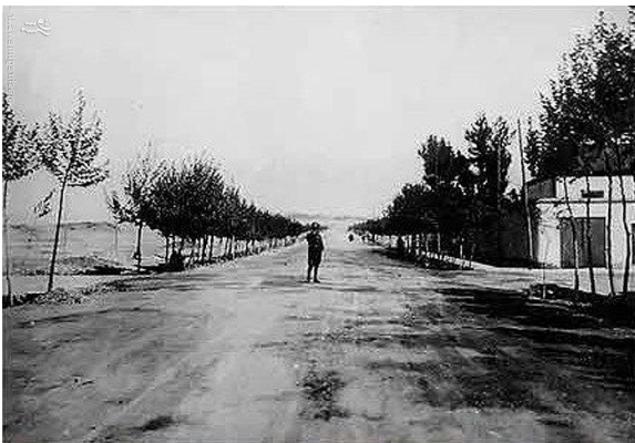
Picture 1. Vali-Asr Street Under Construction
