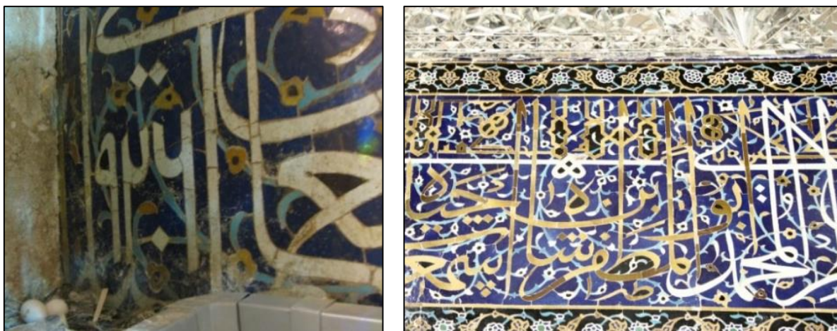
Figs 6-7. the inscription of the entrance porch to the surrounding archway - on the eastern side of the shrine, dated 926 AH known as the Ivan of Shah Ismail. There are Pictures of the current situation and the image that is related to the wainscots before digging and replacing them with stone.
