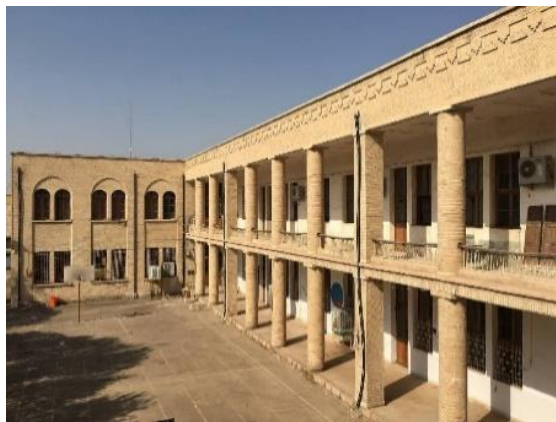
Fig 25 to 27. Hakim Nezami High School in Qom (of course, in the guide of Qom, 1938, it is called Hekmat). The above pictures in the guide of Qom (1938) were taken during the construction of this building, and the scaffolding and materials show the use of old execution techniques in this building with a jack-arched roof. The arches used in this building are not only decorative but also fully load-bearing. The image below shows the contemporary condition of this building. (Qompajoohi, 2021) ("Guide to Qom," 1938)
