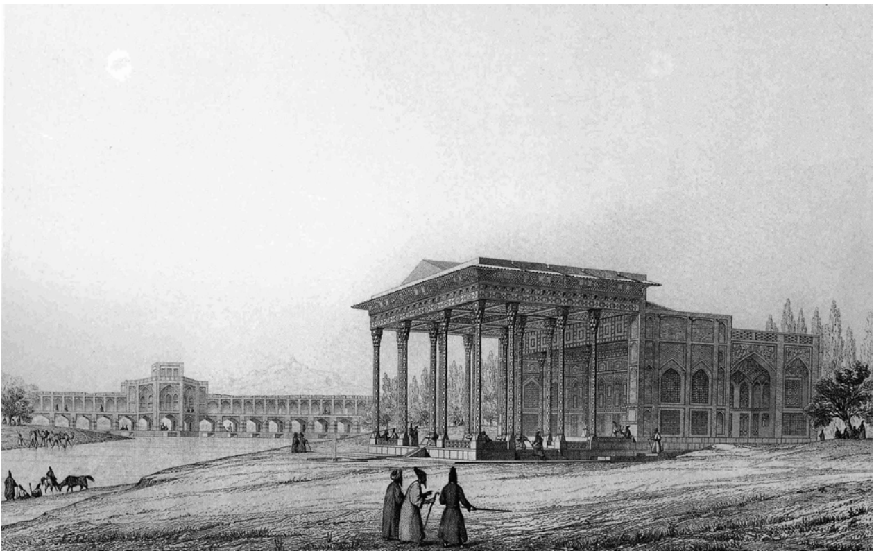
Fig. 3 Khaju Bridge and a part of Saadat-Abad Garden in the Seventeenth Century [16]
