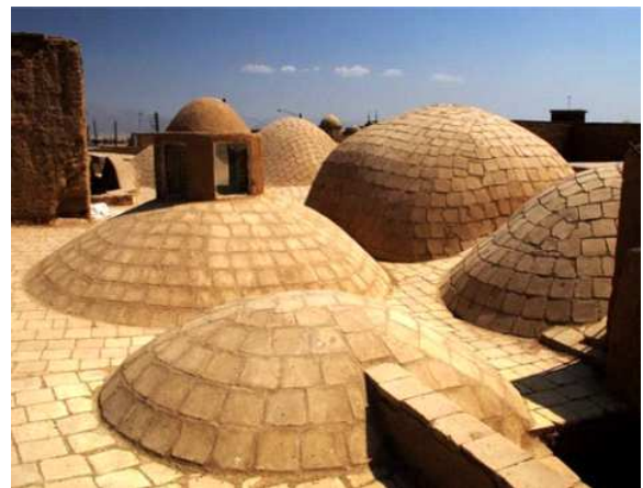
Fig. 5. The dome roof
