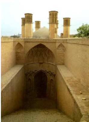
Fig. 11. six wind catcher Abanbar in Yazd
