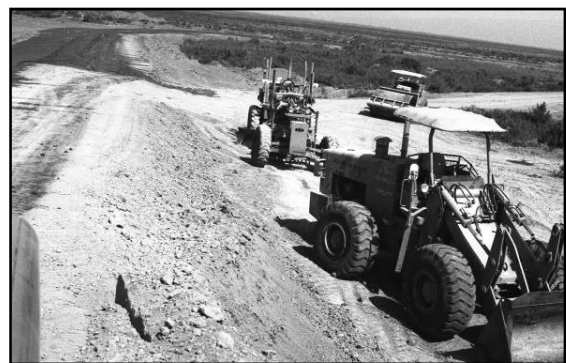
Fig. 4. Using heavy machineries to remove debris and surface the town (Authors)
