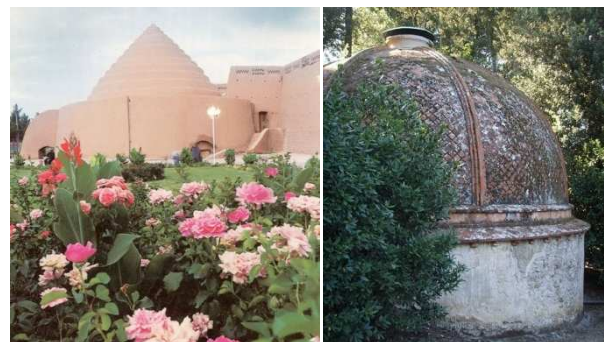
Fig. 14. a) An ancient ice house, called a Yakh-chal, built in Kerman, Iran during the middle ages, for storing ice during summers. b) Boboli Gardens, Florence: domed icehouse (ghiacciaia) half-sunk into a shaded slope.
