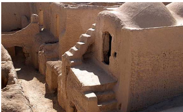
Fig. 7. High thermal mass works well in hot desert climates [14].
