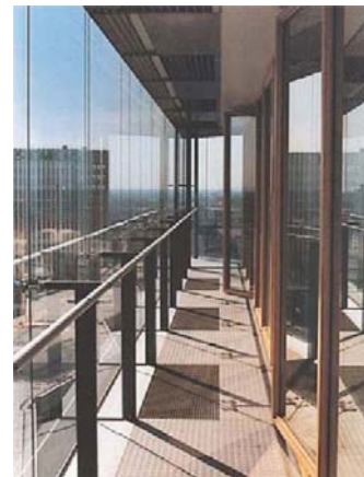
Fig. 5 View of double skin façade of Duesseldorf City Gate [26]
