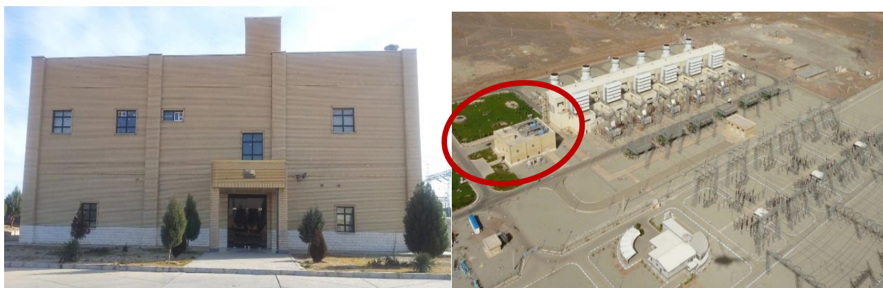
Fig. 2 The picture on the right- the typical control building near the of power plant turbine building, source: URL1 The picture on the left- the façade of the typical control building, source: authors
