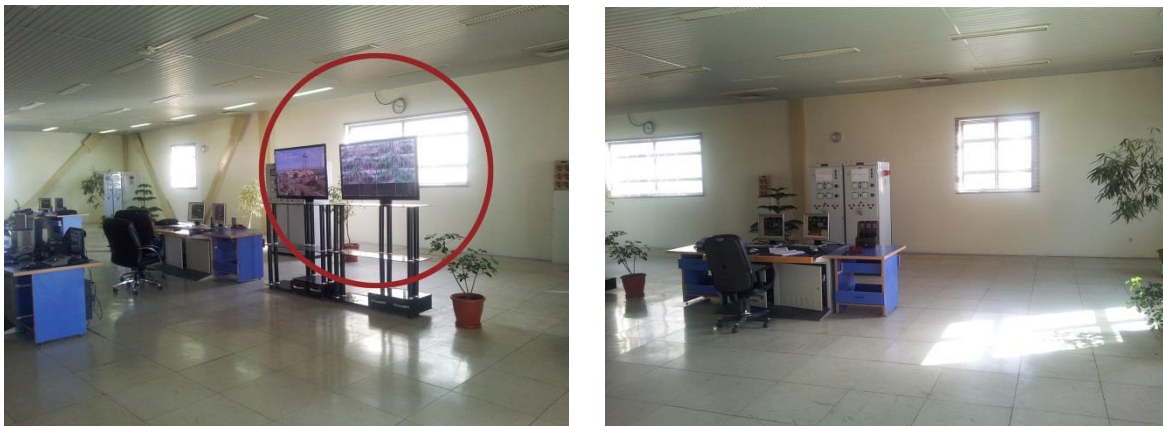
Fig. 5 The photo on the right- control room has a false floor covered with anti-static vinyl tiles. The reflectivity of flooring has tremendously reduced visual quality of space
