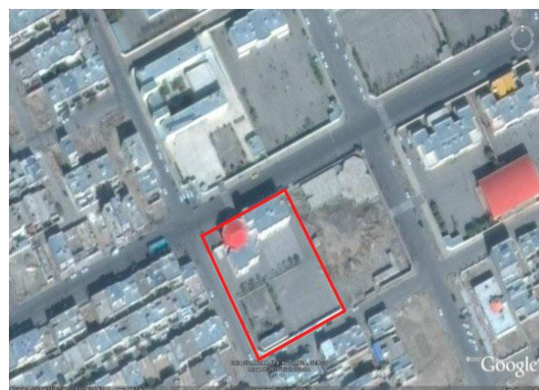
Fig. 1 Top view of the school building
