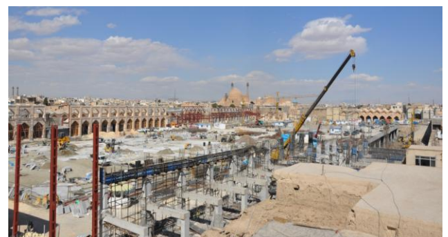
Fig. 4 The Atique square under construction (2012)
