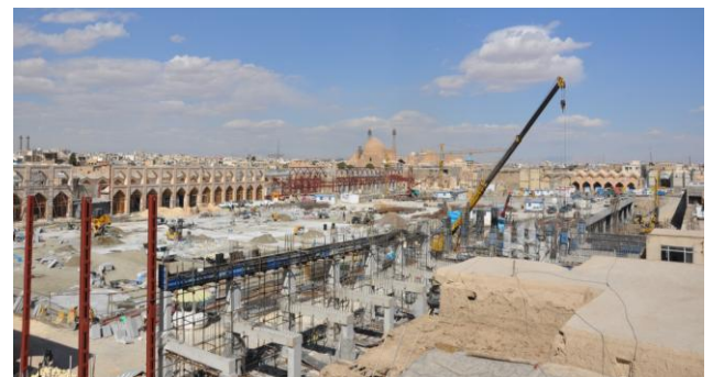
Fig. 4 The Atique square under construction (2012)
