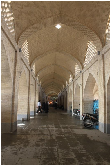
Fig. 5 The revitalized Isfahan Bazaar at the former intersection with Abdolrazagh Street (2012)
