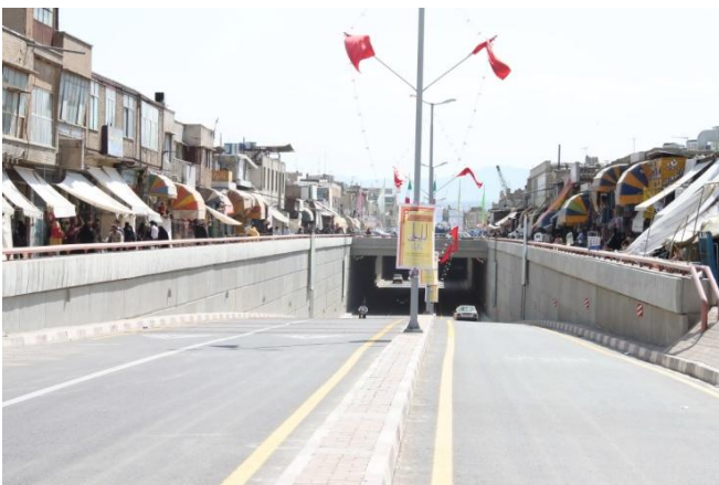
Fig. 3a Abdolrazagh Underpass axis, (2012)
