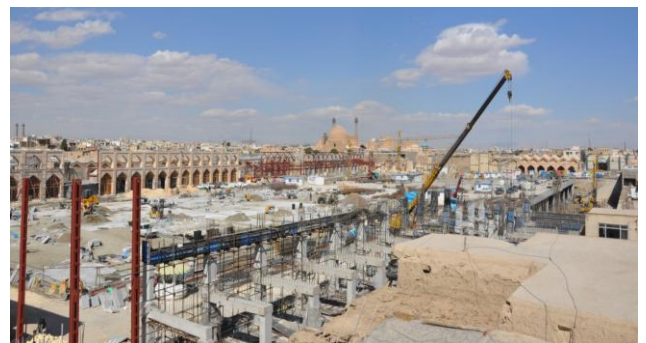
Fig. 4 The Atique square under construction (2012)
