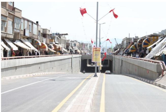
Fig. 3a Abdolrazagh Underpass axis, (2012)
