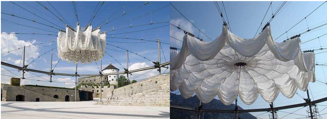
Fig. 4. The retractable membrane roof over the Fortress Kufstein Courtyard in Austria [9]
