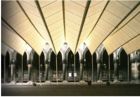
Fig. 3. Roof over the courtyard of Vienna in closed and open positions [8].
