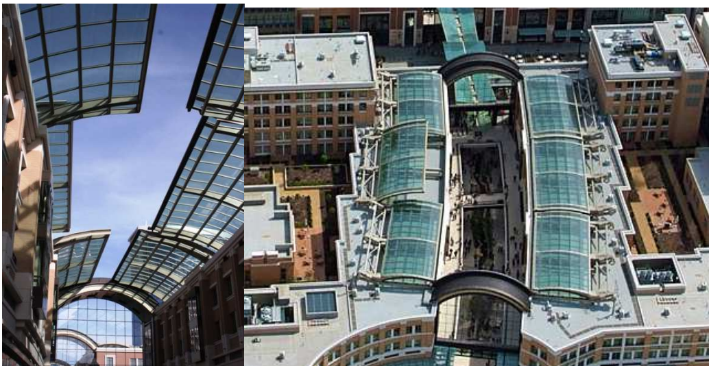
Fig. 2. Retractable sliding roof over the City Creek Centre (Photos Courtesy of Uni-Systems)
