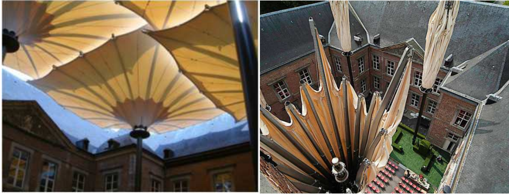
Fig. 1. Retractable umbrellas over Alden Biesen courtyard in Belgium [5]
