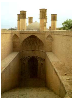
Fig. 11. six wind catcher Abanbar in Yazd
