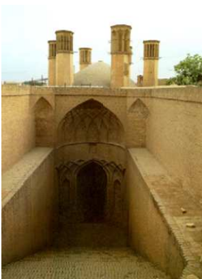
Fig. 11. six wind catcher Abanbar in Yazd
