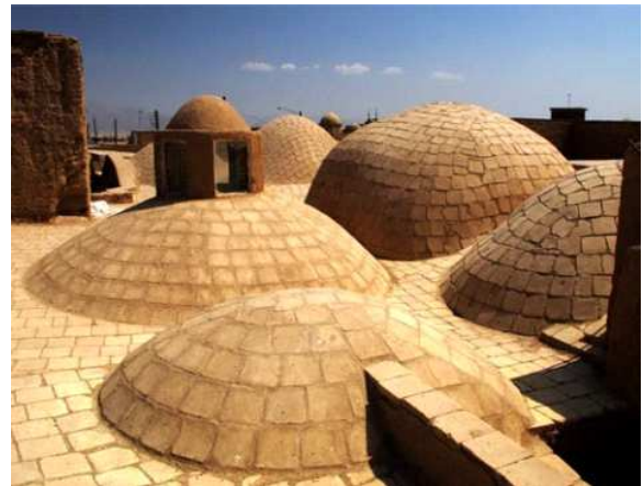
Fig. 5. The dome roof
