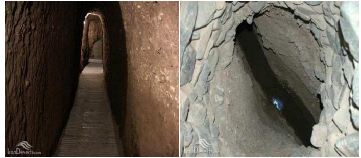
Fig. 10. Shafts, Manholes and Tunnel of Qanat
