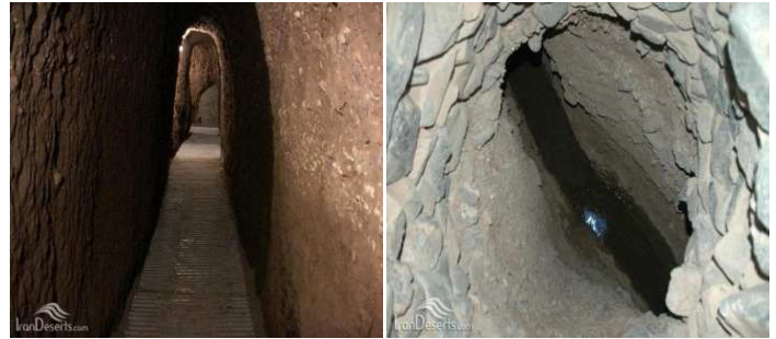
Fig. 10. Shafts, Manholes and Tunnel of Qanat
