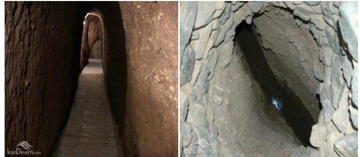
Fig. 10. Shafts, Manholes and Tunnel of Qanat
