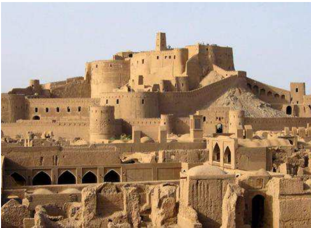
Fig. 1. The Citadel of Bam, before earthquake.
