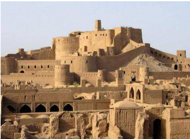
Fig. 1. The Citadel of Bam, before earthquake.
