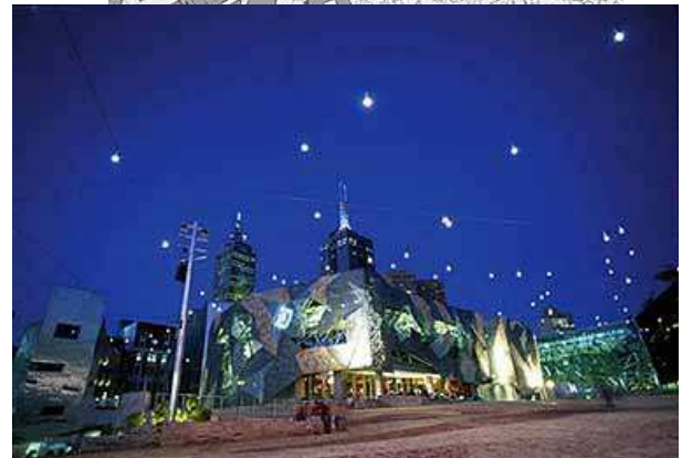
Fig. 9 & 10. Federation Square and complex of buildings (the Australian Centre for the Moving Image (ACMI), SBS (Australia's multi-cultural broadcaster), Melbourne's Visitor Information Centre) designed by LAB Studio has given a new character to the urban landscape near Yarra River [9]
