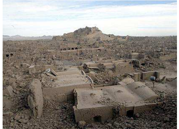
Fig. 2. The Citadel of Bam after earthquake. http://explo.com/2003_Bam_earthquake
