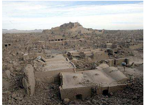
Fig. 2. The Citadel of Bam after earthquake. http://explo.com/2003_Bam_earthquake
