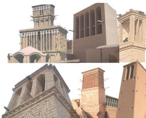
Fig1: Wind towers in Iran [Authors]
