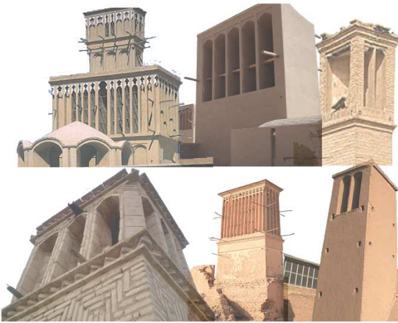
Fig. 1. Wind towers in Iran [Authors]
